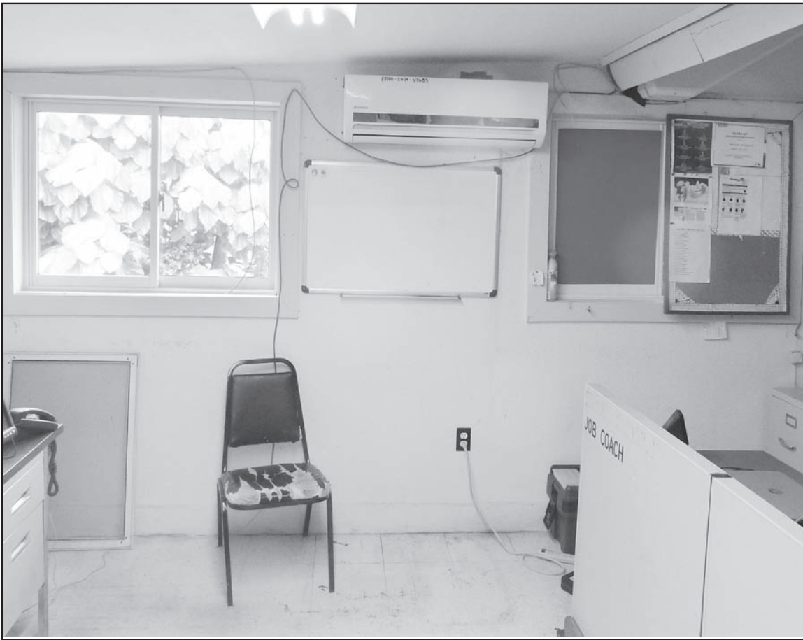
This Samoa News photo taken on Mar. 30 shows the already repaired back window at the Vocational Rehabilitation (or Voc Rehab) Office building at the government housing complex in Tafuna, across from the Pala Lagoon park.
