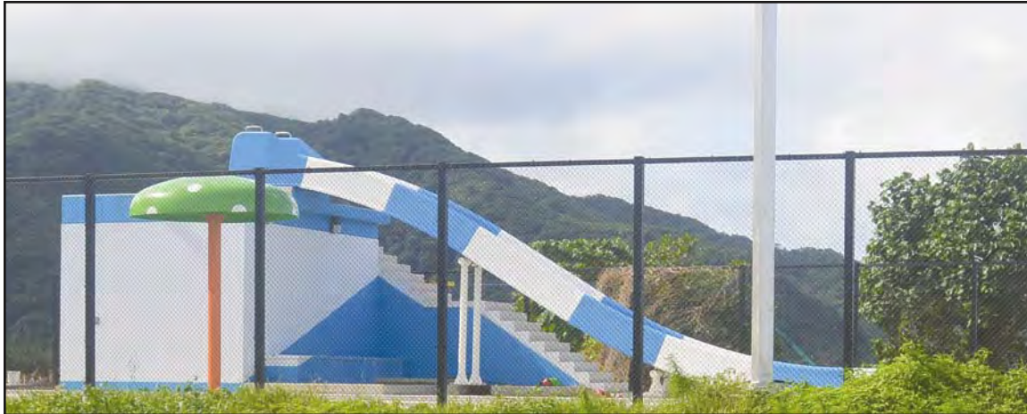
A look at the Pala Lagoon Swimming Center while still being constructed. It is set to open today, after 15 years in the making. See story for details. [SN archives]
